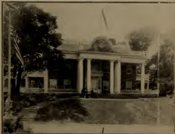
Rhode Island Building
